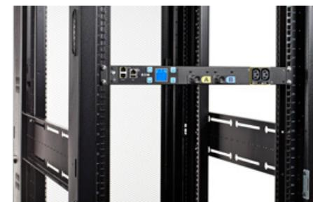
Here is an example of a horizontally-mounted 1U PDU.
